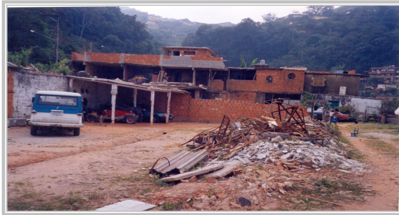
Build on top of the hill and embankment area.
