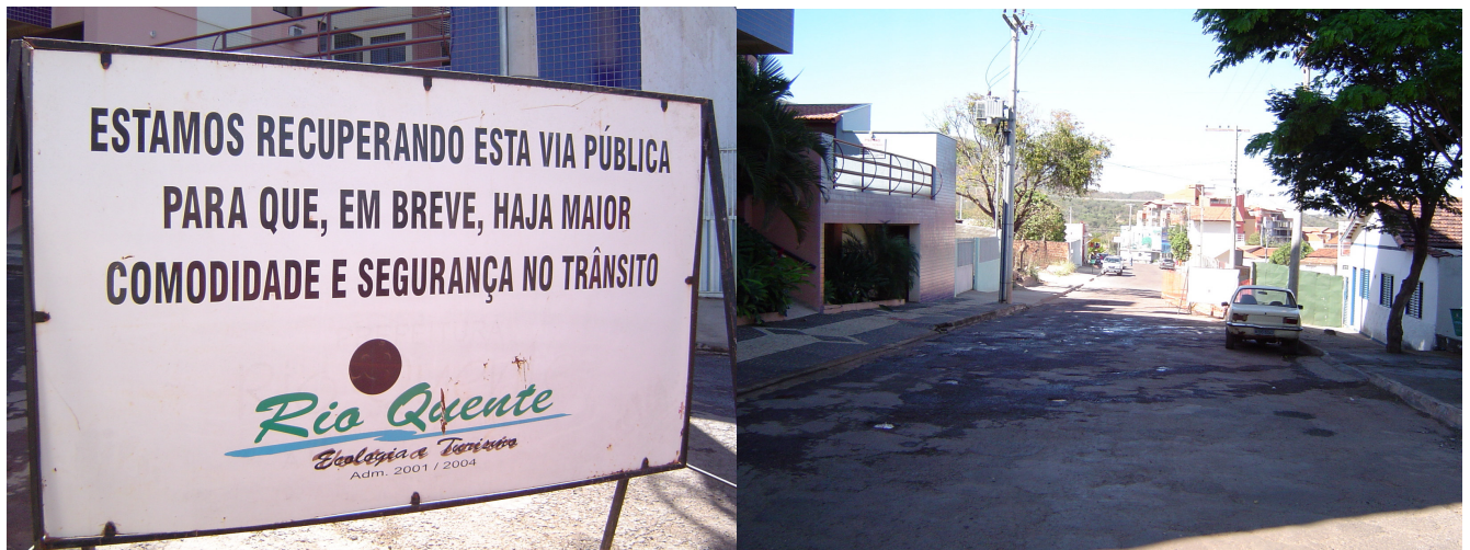
Pavement of a street being arranged by Pousasda do Rio Quente
