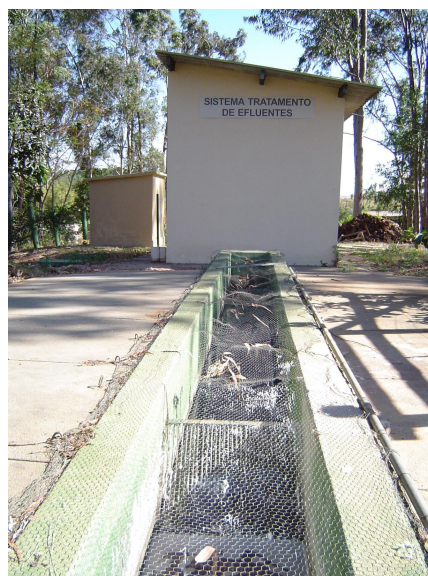
Partial vision of the Station of Treatment of Effluent of the laundry
