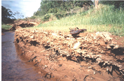
Sediment deposited in lake
