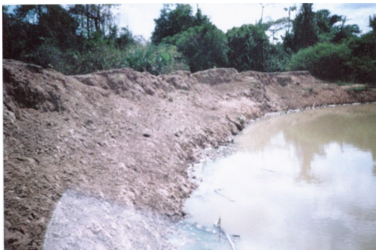
Picture 05 – Erosion on the riverbanks
