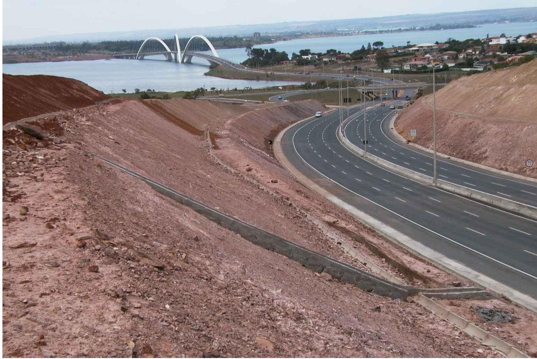
Figure 3 - Sight of cut slopes in highway EPDB/EPCT after concluded the pavement services.
