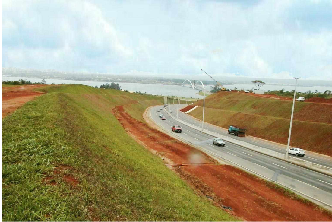
Figure 11 - Conclusion of the work.
