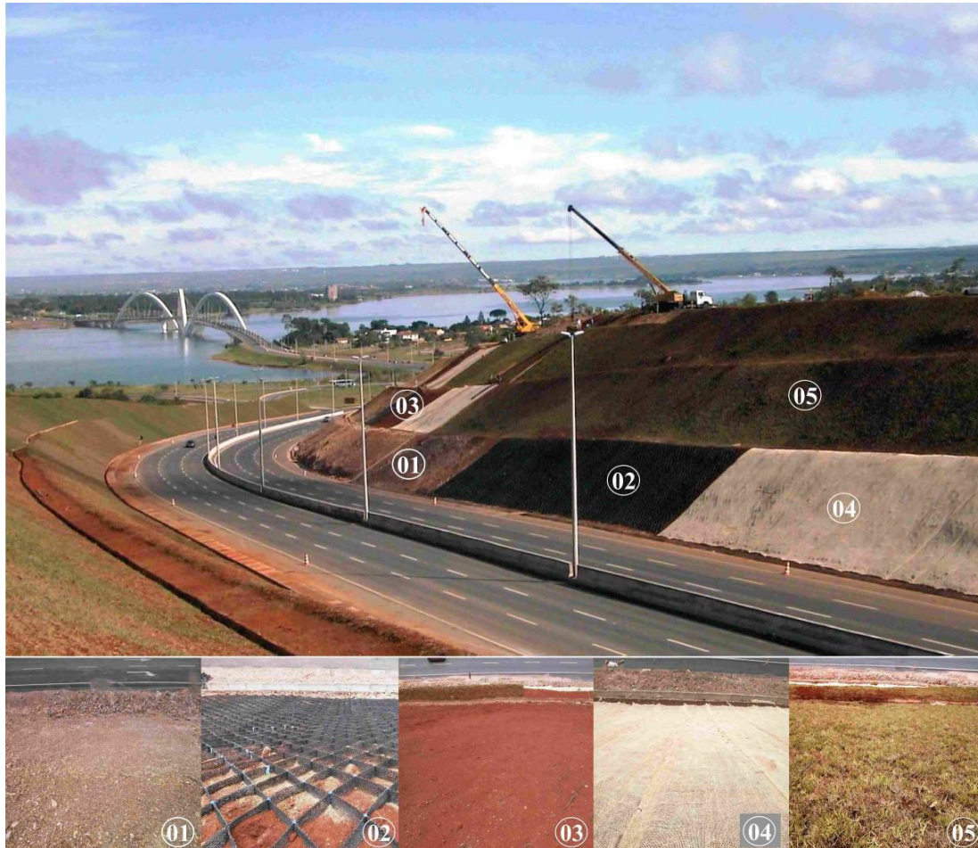
Figure 10 - Synthesis of the stages of implantation of geocells and plantation of grass: 1) regularization of slopes; 2) implantation of geocells; 3) filling with top soil; 4) application of bioblanket in sisal; e 5) plantation of grass.
