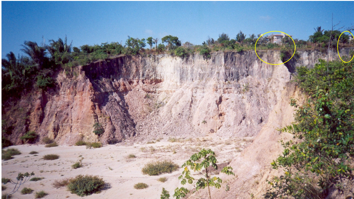
Figure 3: Paço do Lumiar city's gully: Note the presence of houses at the top of the photo, threatened by the progress of the gully (Photo: Sathler, 2004)
