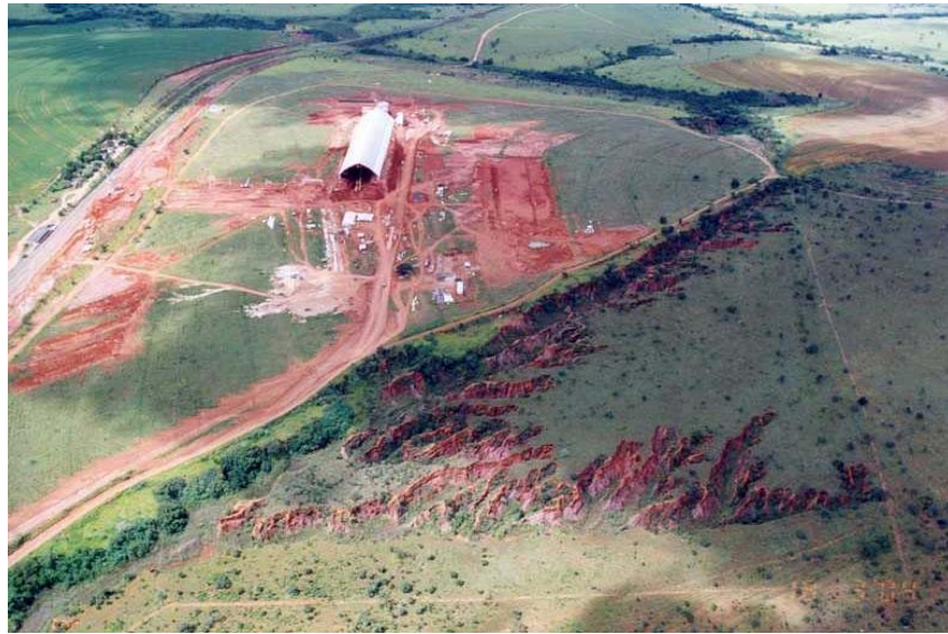
Fig.1 – In this picture it is possible to see the erosion process where this paper have being developed. Also, it is possible to make a comparison between the size of the facture (at the bottom of the picture) and the gully studied located at the front of the picture (ROCHA, Erica – 2004).
