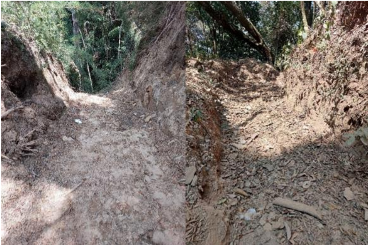
Figure 7 – Rustic drainage systems
