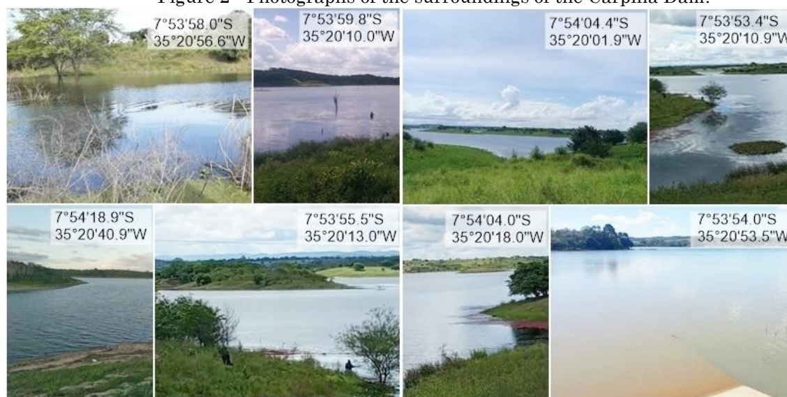
Figure 2 - Photographs of the surroundings of the Carpina Dam.
