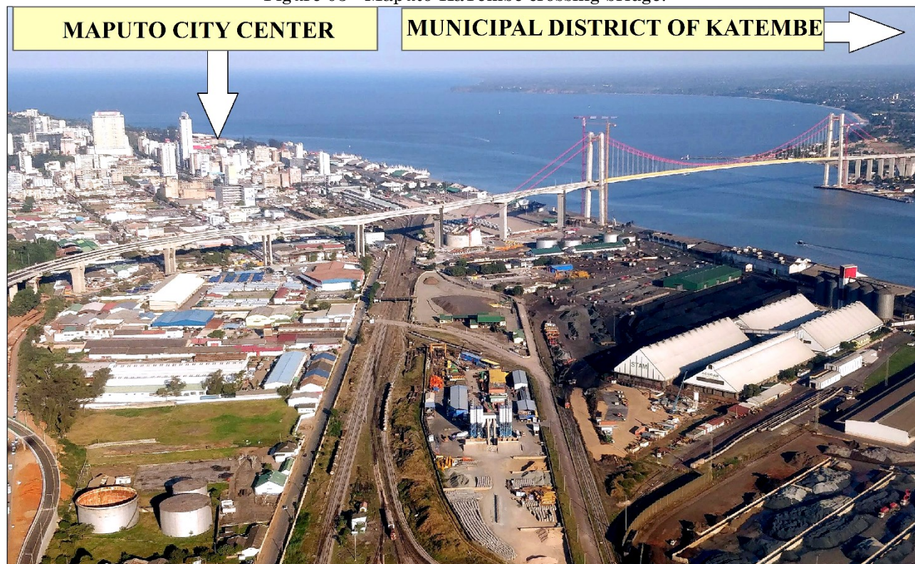
Figure 03 - Maputo-KaTembe crossing bridge.
