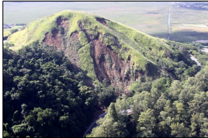
Figure 9 – Grota Funda Rd. landslide gullies, April/2010
