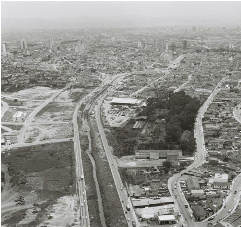
Figure 4 – An aerial view of the works for the opening of Avenida Água Funda (now Av. Dr. Ricardo Jafet), and the rectification of the Ipiranga Stream, in the section that cuts through Vila São José neighborhood. View taken towards Vila Monumento neighborhood, 1970, São Paulo/SP.
