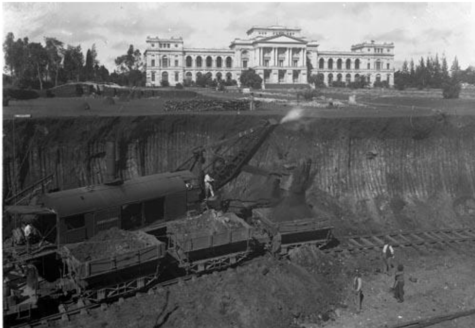
Figure 3 – The works for rectification of Ipiranga Stream (1910-1920) In the picture in the background is the Paulista Museum, popularly known as the Ipiranga Museum.
