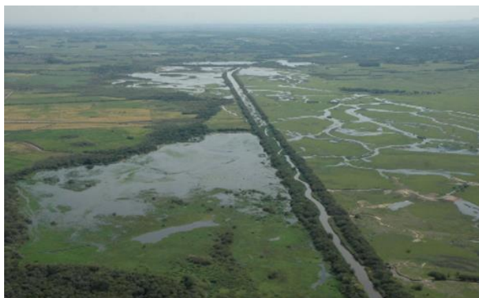
Figure 2 - Wetland in the Environmental Preservation Area (EPA) of Banhado Grande.
