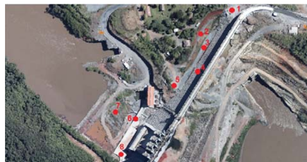
Fig. 4 - Approximate locations of the points in the TLS survey
