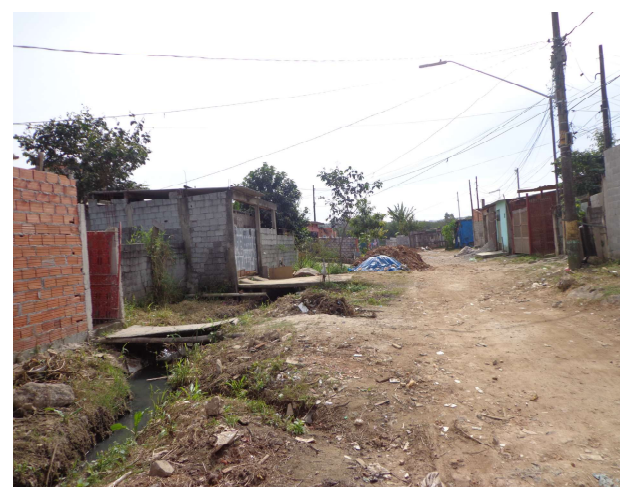
Fig. 5 - Open sewage and unpaved street.
