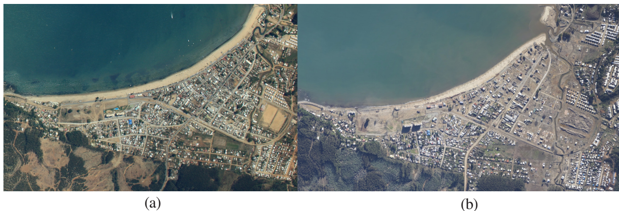
Fig. 3 – Dichato, Chile, before (3a) and after (3b) the February 27, 2010 tsunami.
