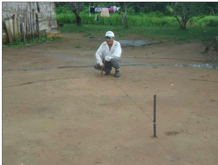
FIGURE 2: Circumference on the ground in the construction of a traditional maloca.
