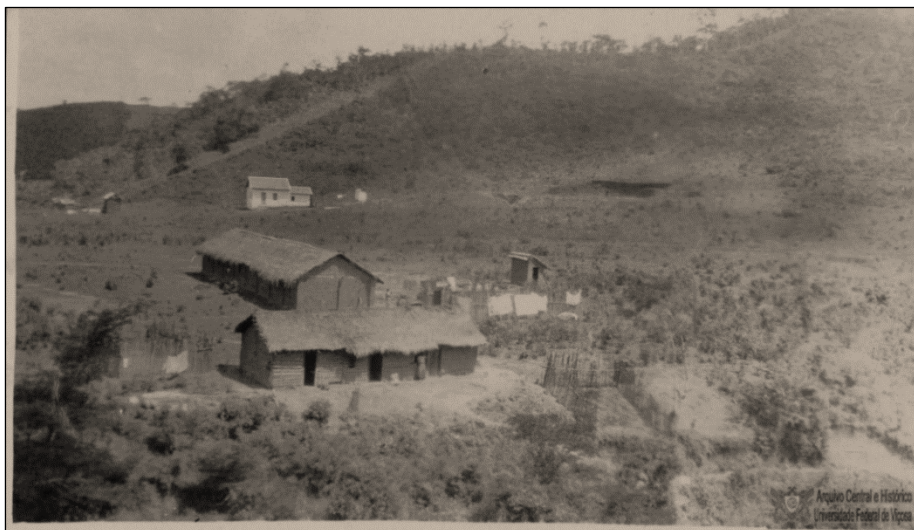
Figure 5 - Housing of the workers who built the School, made of adobe and pau-a-pique (1922). The presence of septic tanks can be seen in both the front and back huts.
