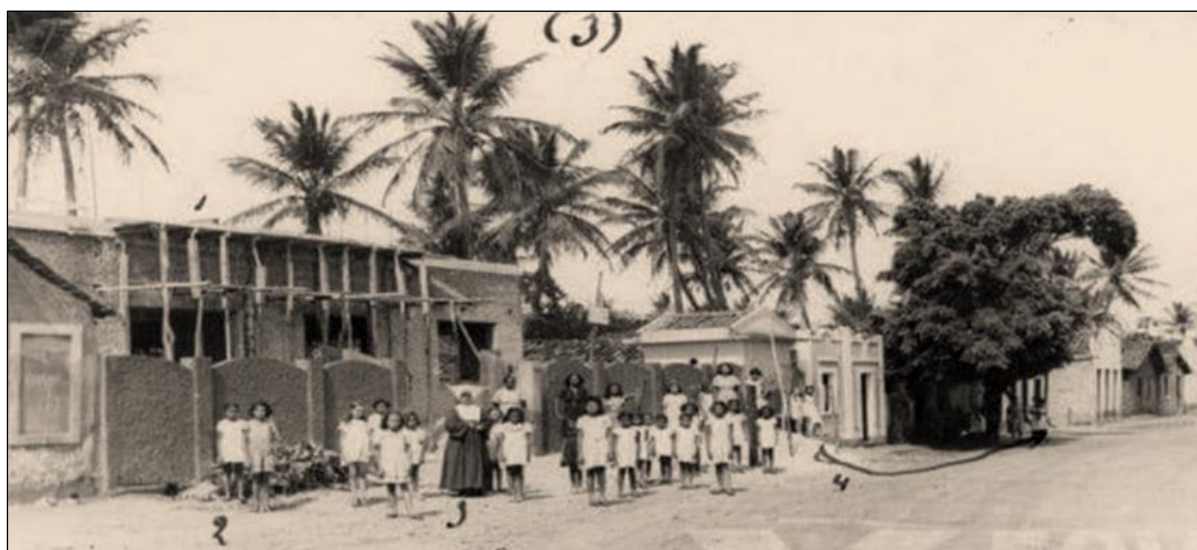
Figure 1 - Beginning of construction of the São José School and Laboratory, led by Sister Vitória, in Rocas
