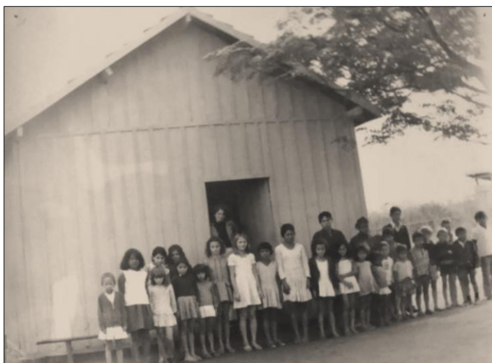
Figure 1. Batayporã School Group Building, backyard (1957)
