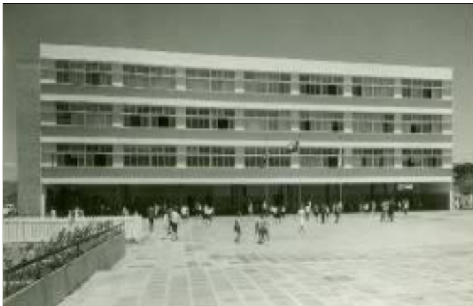
Figure 14: Farroupilha School in the Três Figueiras district.
