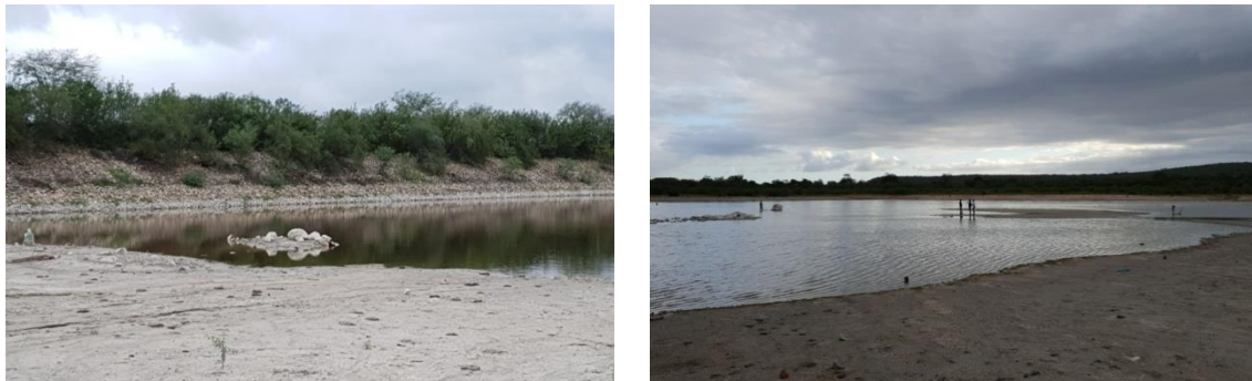
Figure 8 - Açude do DNOCS (1946) in Delmiro Gouveia.
