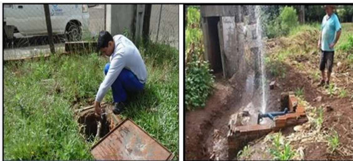
Figure 2 - Deep tubular wells surveyed.
