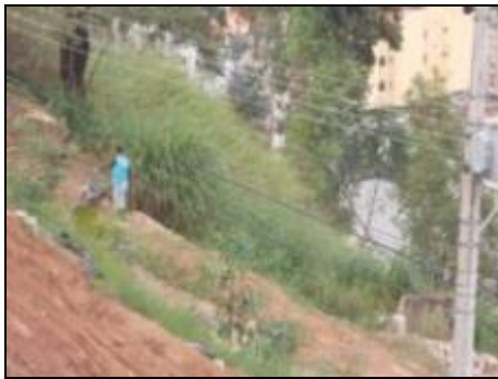
Point 05 - Trash and debris launched on top of the slope
