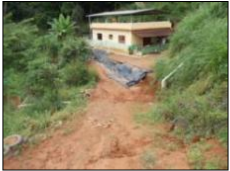
Point 92 - Subsidence caused by margin erosion, on a creek
