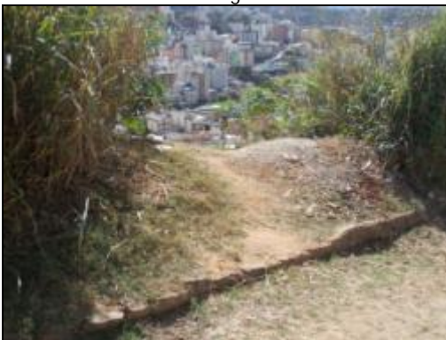
Point 12 - Disposal of dump on top of a slope
